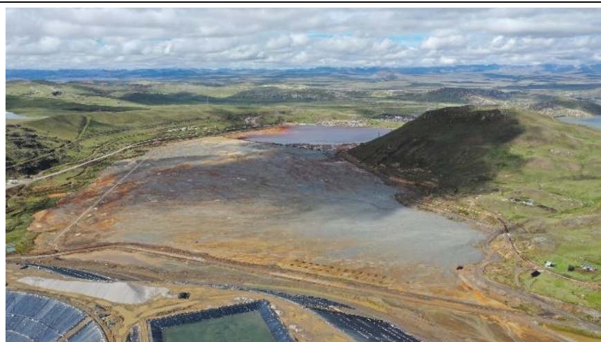
Quiulacocha TSF, potential reprocessing target (looking southwest)
